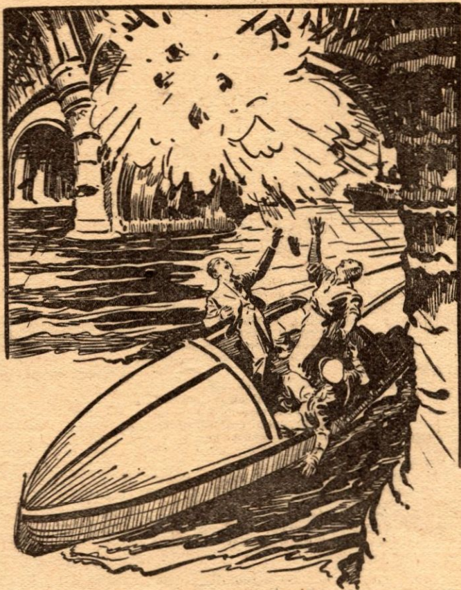
THE BRIDGE BOMBARDED.—Billy and Fritz had reached the bridge when a shell hit it. Twisted steel and smashed roadway flew in all directions, and the boat heeled over.
