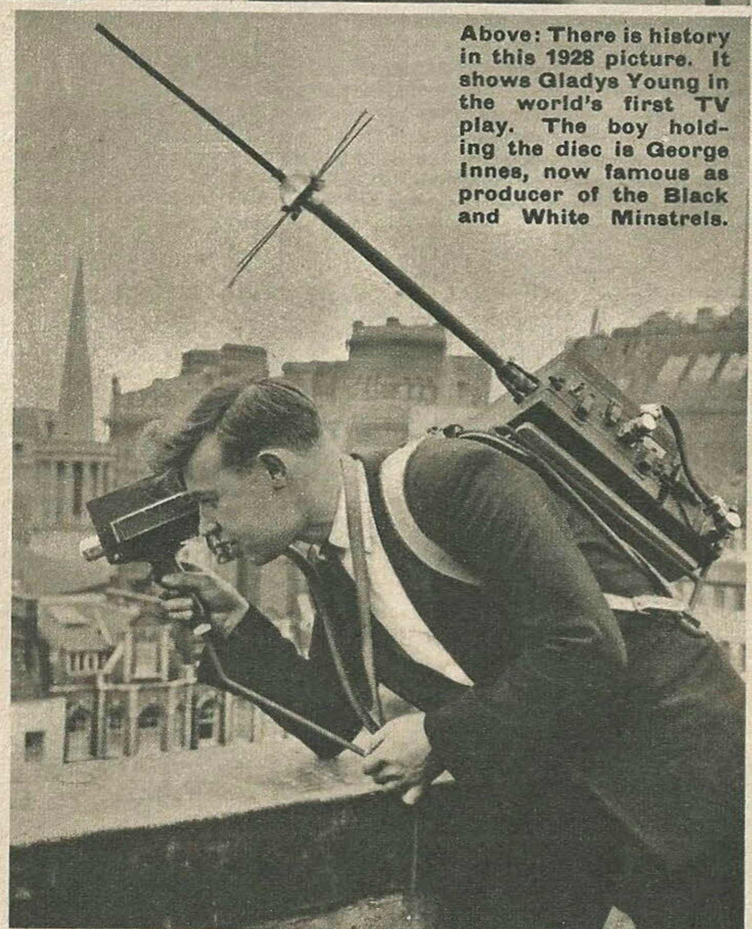
Specially useful in outside TV broadcasts is this one-man TV station. The camera is a midget, and a complete transmitter and aerial are strapped to cameraman's back.
