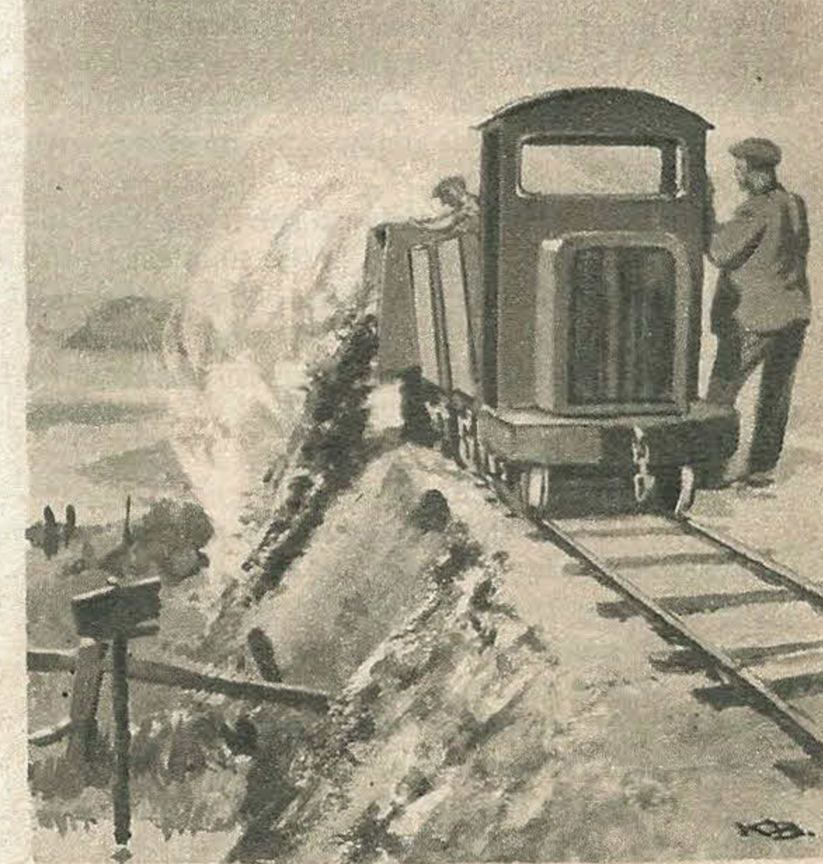
What becomes of the refuse collected? Some of it is burned, some is taken away and tipped on to low-lying marshland, to raise the level of the ground and make it suitable for building upon later. The refuse is sealed in with layers of earth.
