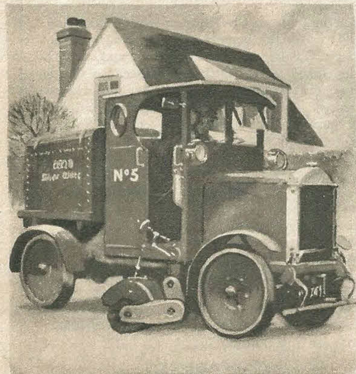
When better roads were laid, with tar macadam surfaces, dust was greatly reduced. But cleansing was still necessary and mechanized vehicles like the one above both watered and swept the streets, brushing the dirt into the gutter.
