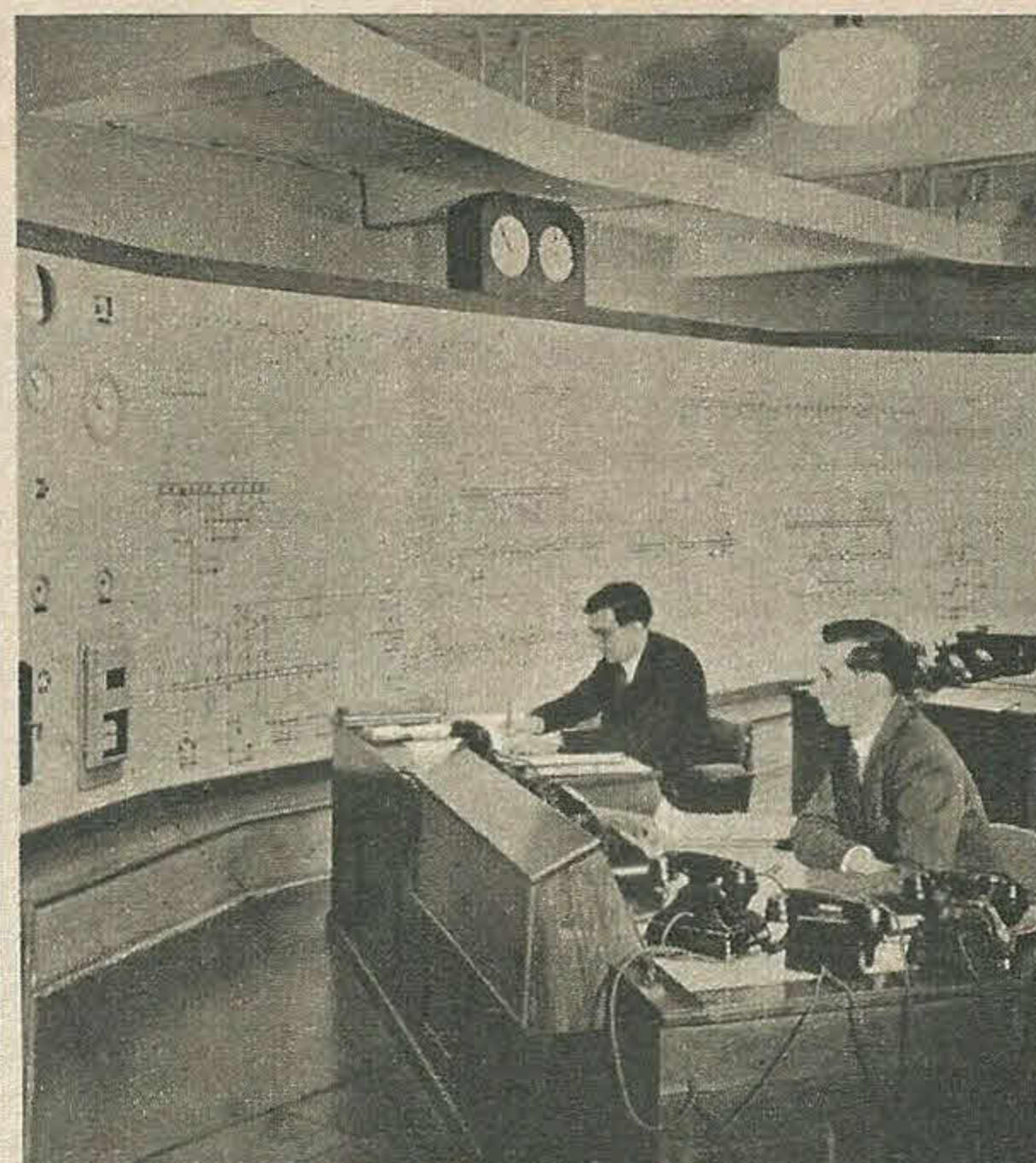
Left: By pressing switches on the right of his cabinet, called a console, the supervisor at an oil depot automatically loads a fleet of road tankers. When each tanker is full, a lamp lights. Robots hidden by the great wall diagram in the top photograph tell controllers at an electricity distribution centre how power is being used.
