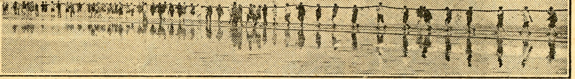
The "sea-serpent" coming ashore! Man-handling part of a 70 miles long cable.
