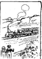
Stephenson became the principal builder of railways in Britain, and here we see one of his first engines hauling the first passenger and goods trains on the Stockton and Darlington Railway at its opening in 1825. Steam in railway travel had yet to be developed.
