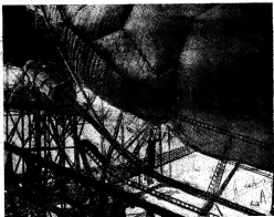
You see from this photo how the enormous gangway of the sturdy R.M.S. are attached to the frames. Note the workman standing on one of the girders. That will give you an idea of the general proportions of this wonderful ship of the air. (See opposite page.)
