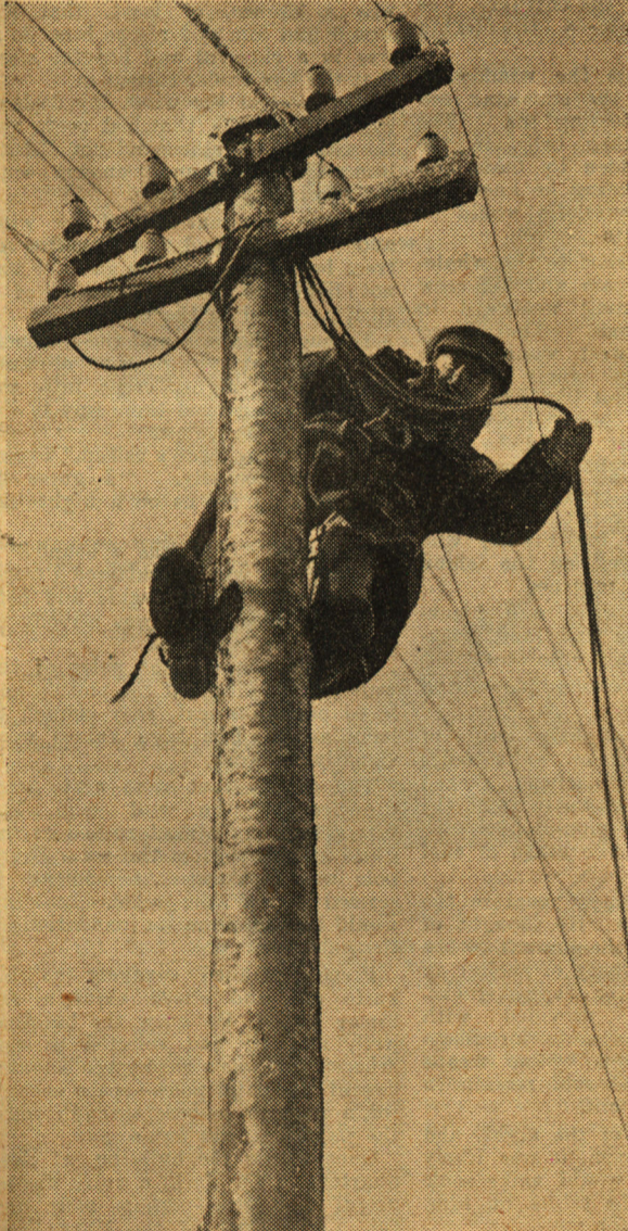
A G.P.O. linesman, perched precariously at the top of a telegraph pole, mending broken wires in a mile-a-minute gale!
